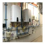
High-end custom homebuilder Hickory Construction offers tankless water heaters as standard. The company often supplements the tankless units with a small, tanked water heater and ties in a recirculation system to ensure water supply is ample and at a consistent temperature. Visit **Propane.com** to learn how propane tankless water heaters help Hickory keep customer satisfaction high.
