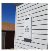
A propane tankless water heater helped California builder Steve Lefler design his home to the state's forthcoming net-zero energy standards well ahead of the compliance deadline. A 3 kW photovoltaic system provides nearly all of the home's needs — except for water heating. But instead of installing a larger solar array to handle that demand, he simply turned to a propane tankless water heater. Visit **Propane.com** to learn how propane helped Lefler build net-zero.
